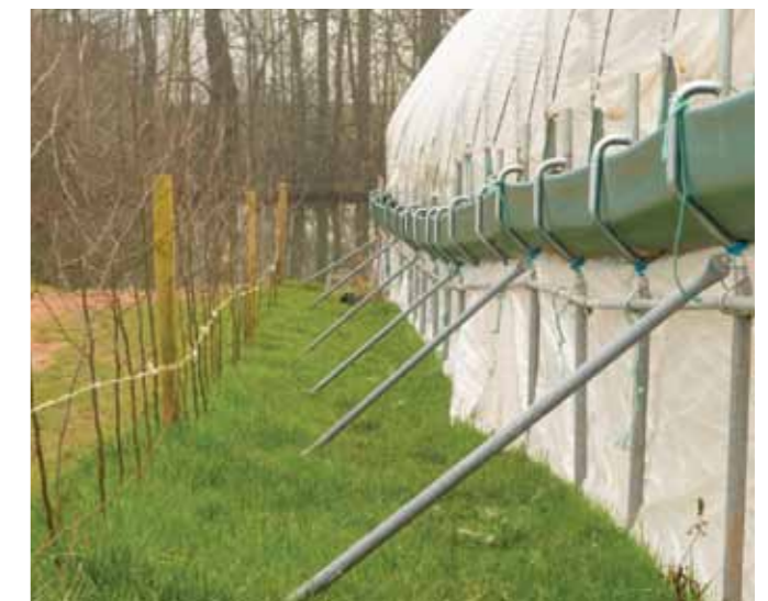
Harvested rainwater is collected from polytunnels in the guttering shown and then collected in the lined reservoir to be used for irrigation
