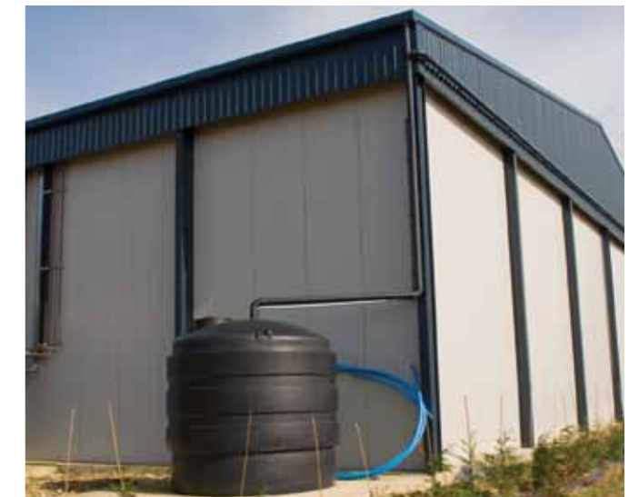
The amount of rainfall that can be collected depends on your roof area
