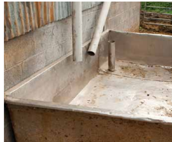
Roofwater enters the drinking trough and a level overflow takes it to the surface water drains
