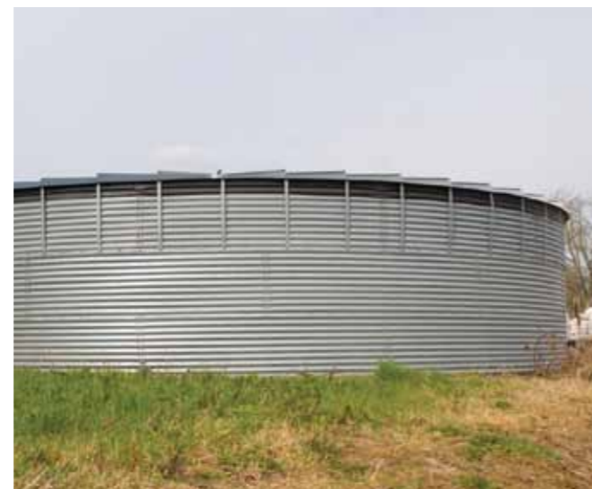
A new large above ground store
